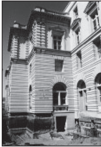
Figure 1 View of U.S. Court of Appeals Building in San Francisco, California, isolated with friction pendulum bearings
